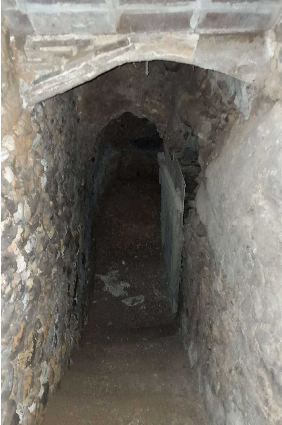
Vista escala existent PB a PS.
