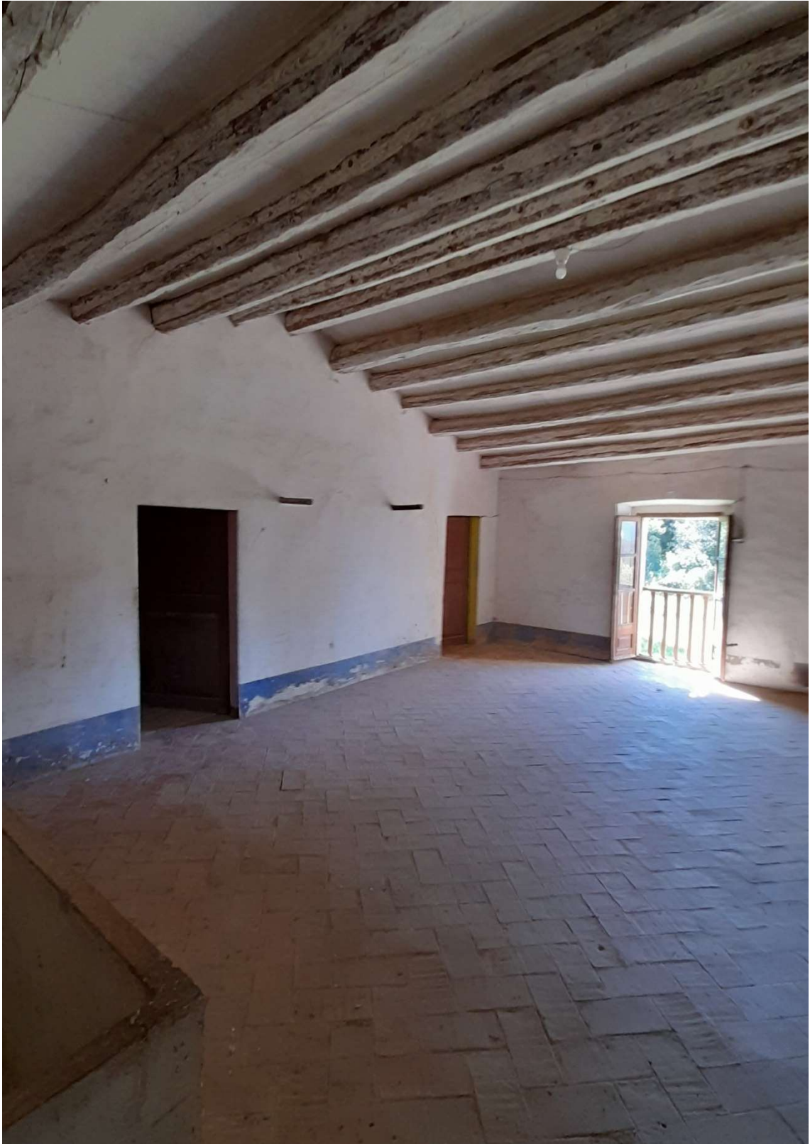
Vista crugia central P1.
