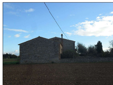
VISTA GENERAL OEST
