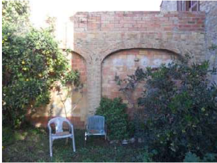
Annex Oest (arcs carpanells)
