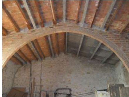
Arc interior (Annex Oest)
